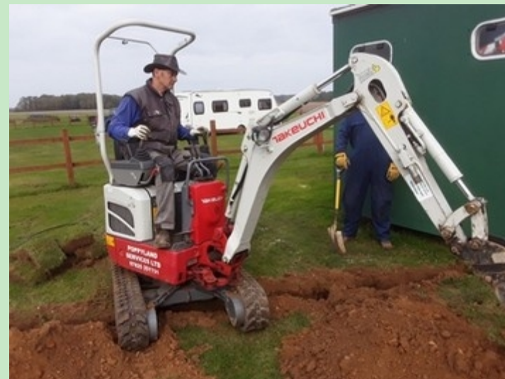
Mike digging the last metre to Air Traffic Control
